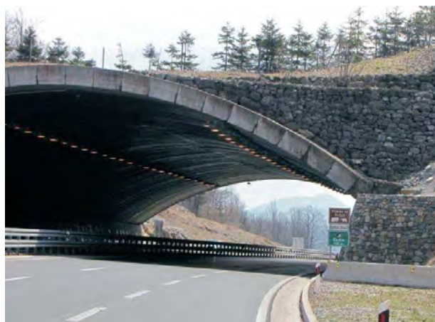
Figure 71. Large overpass (green bridge) of 120 m wide on Highway A6 in Croatia (Jedrzejewski 2009).
