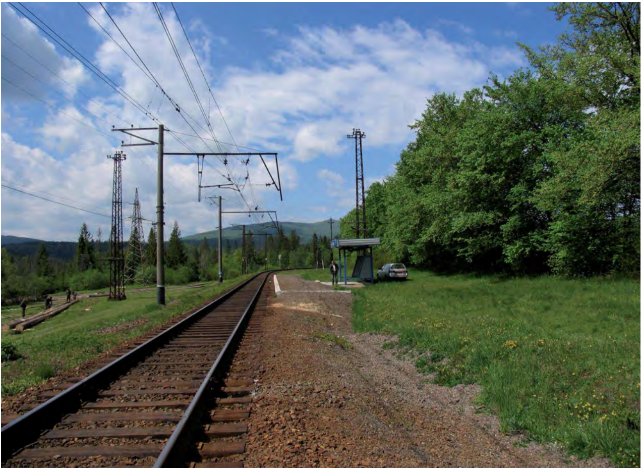
Figure 49. Railroads of low frequency use do usually not intervene much with connectivity.
