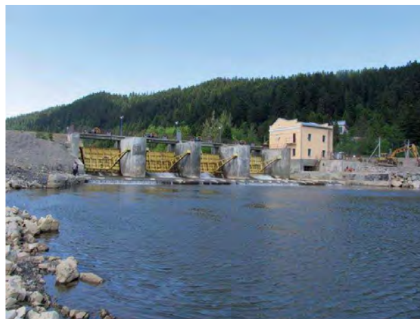
Figure 69. Dams intervene with connectivity in two ways: they are an absolute barrier for aquatic species, but water level rises and lakes associated with dams have a serious effect on connectivity for terrestrial animals as well. Development plans for dams should therefore take corridors into account.
