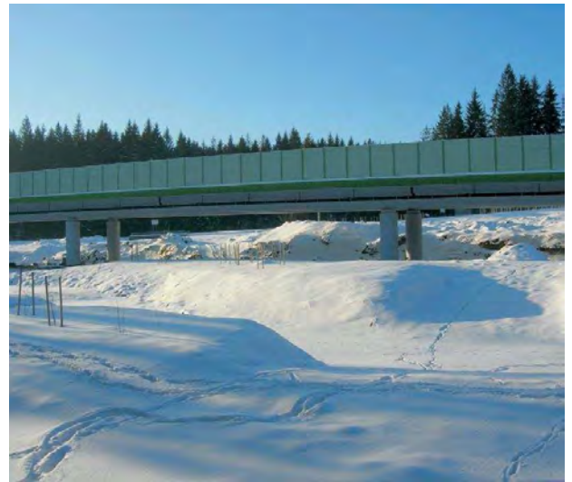
Figure 72. A wildlife passage under a 200 m long viaduct on Express Road S69 near Zwardoń, south Poland. Note the animal tracks in the snow (Jedrzejewski 2009).
