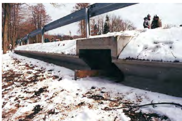
Figure 70. A passage for amphibians on a regional road near Kudowa Zdroj, south-western Poland (Jedrzejewski et al 2009).
